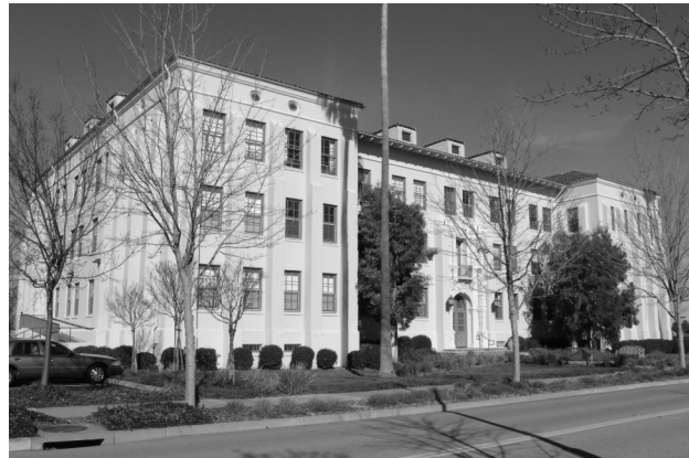
Former officer quarters at Hamilton Air Force Base in Novato have been converted to apartments for seniors.
