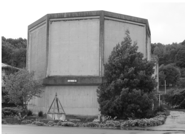
The untreated waste water filling this bio tower at Central Marin Sanitation Agency will be converted into water that can be released into the bay through an organic treatment in which bacteria in the plant eat the waste, or nutrients, in the raw sewage.
